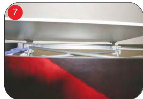
7-8. Install counter tops, inserting hubs securely into routed locations.
